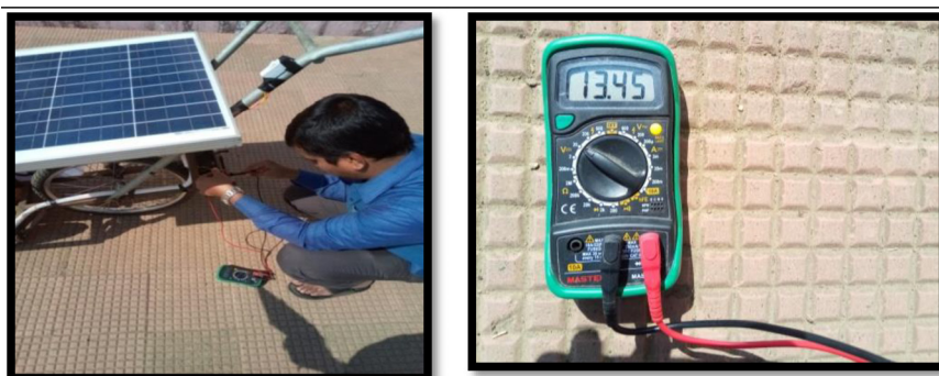
Fig. 7. Testing discharging of battery with multimeter.
